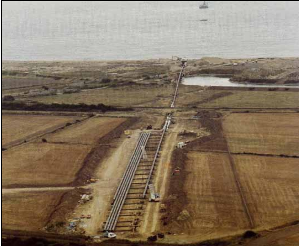
Photograph 9-3 Typical Overview of Pipe String Launching Operation (Several Strings)
