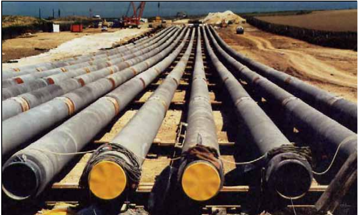
Photograph 9-1 Concrete Coated Steel Pipeline Strings for Long Sea Outfall
