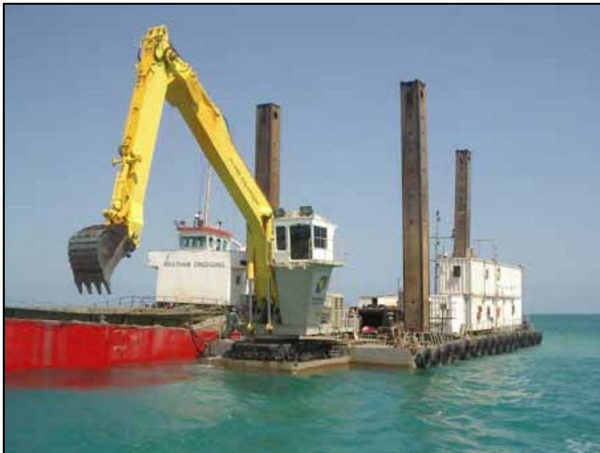
Photograph 9-2 Back Hoe Dredge
