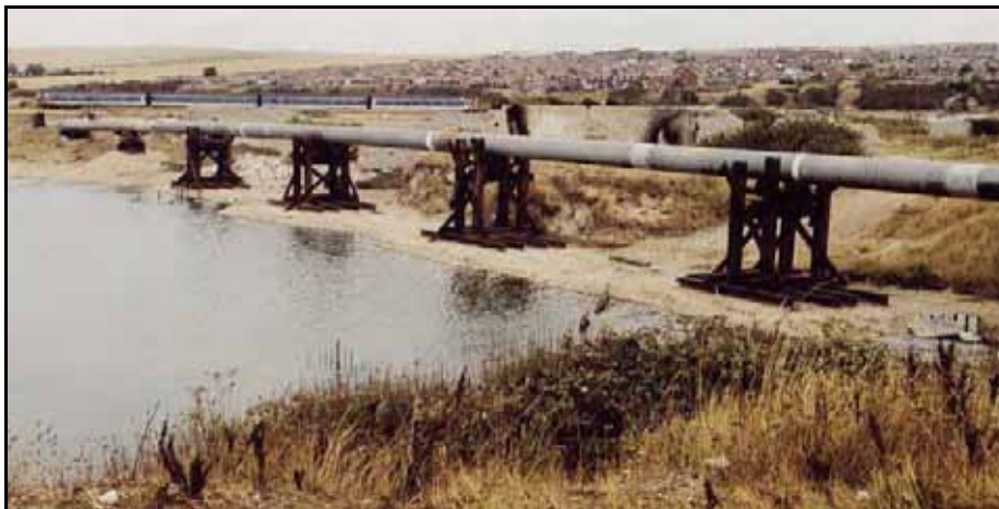
Photograph 9-5 Temporary Tower Supports for 26" Pipe String Launching
